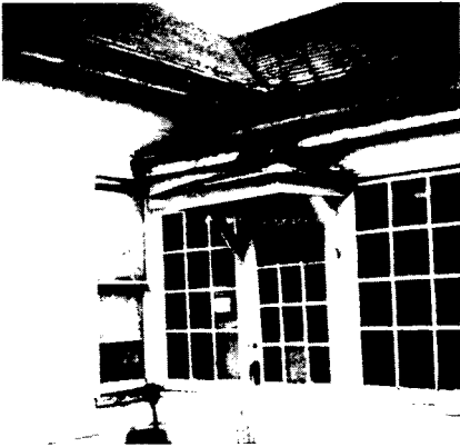
Dilapidated porch, lack of gutters, and warped door. Montesano, Washington.
