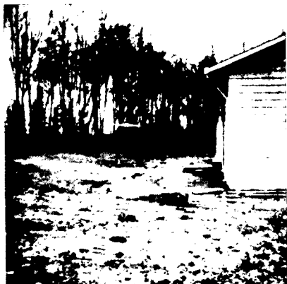
Improper grading resulted in water draining into crawl space; at time of inspection 6 inches of water were under this house. Lynwood, Washington.
