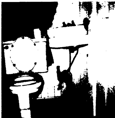
Inoperable bathroom sink blocking a portion of window, Seattle, Washington
